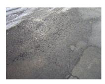
CONDITION: MAINTENANCE: There are cracks and erosion
